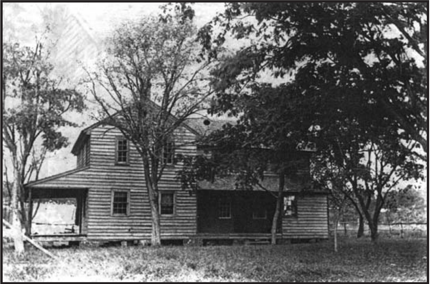
Fig. 2: Meekins Homeplace, side elevation ca. 1915. D. Victor Meekins Collection, Outer Banks History Center, Manteo, NC
