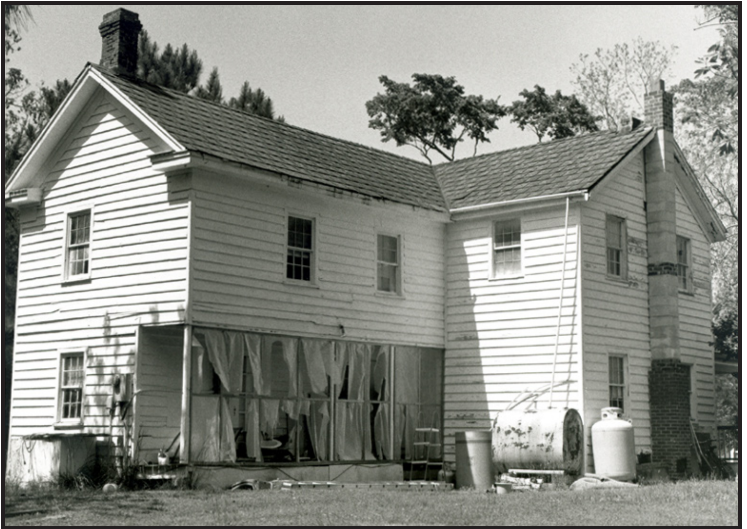
Fig. 8: 1890s rear ell of Etheridge House, May 1999 (Penne Smith, photographer)
