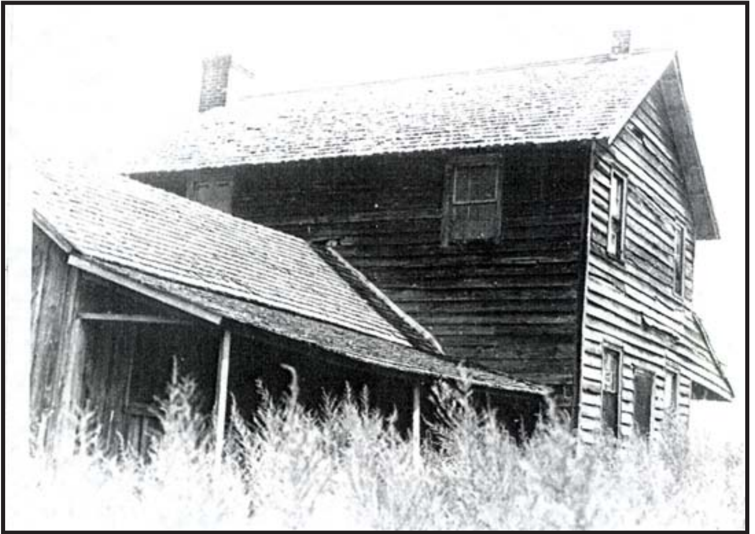
Fig. 13: Dough-Hayman-Drinkwater House, rear and side elevations, ca. 1940. Roger Meekins Collection, Outer Banks History Center, Manteo, NC. N.B. the door surround at the side elevation.
